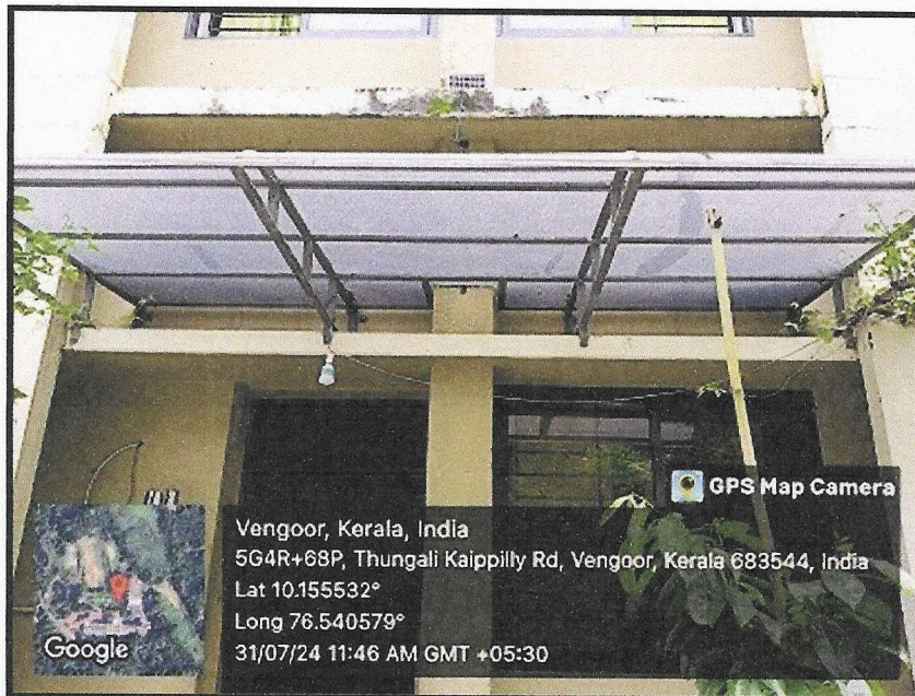
Polycarbonate Sheet Roofing of the Canteen
