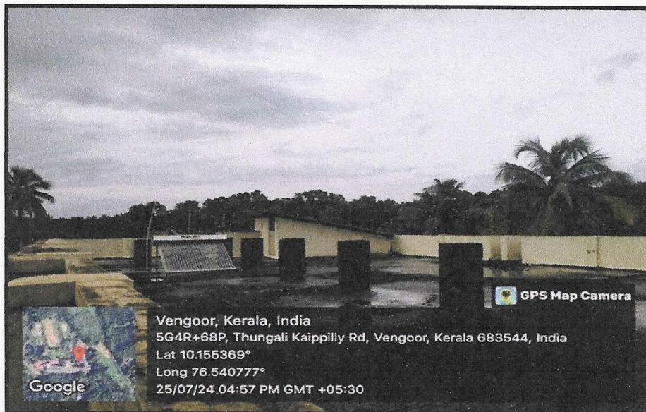
Solar Water Heater Rooftop Installation for the Hostel Building, RVCAS
