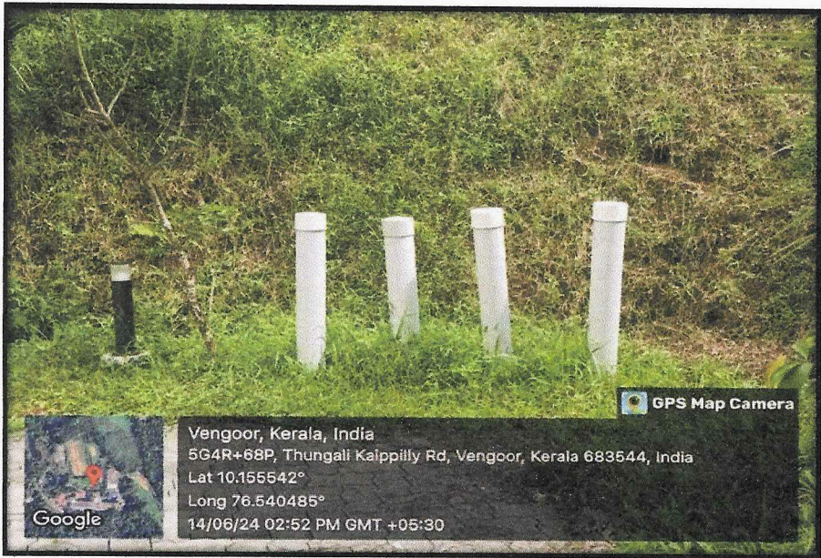
Food Waste Pipe Composting System Near the Canteen
