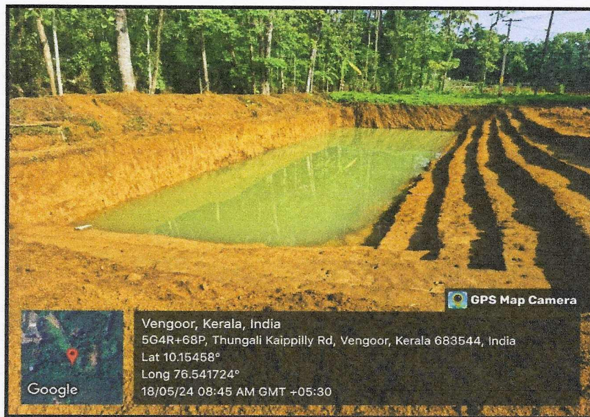
Open Water Recharge Pit
