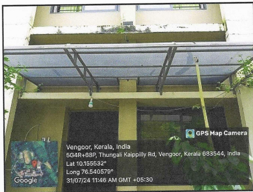
Polycarbonate Sheet Roofing of the Canteen
