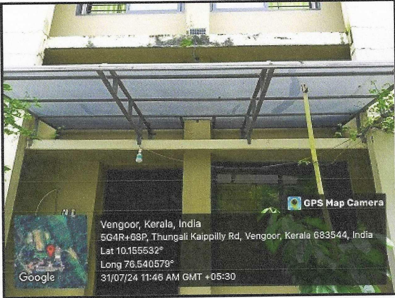
Polyethylene Sheet Roofing of the Canteen
