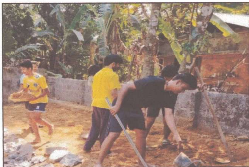
Team NSS Engaging in Construction Process for Snehaveedu Project
